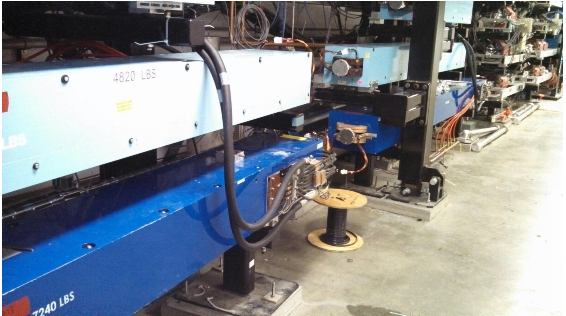
Arc 10 4 meter dipole cable installation
