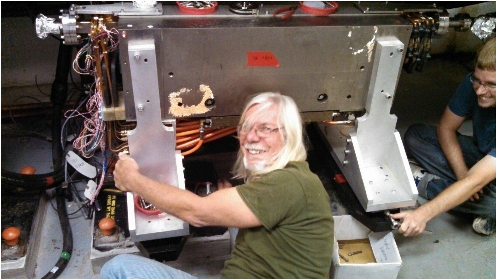
YB Septa Alignment in 1S (obviously happy work...)
